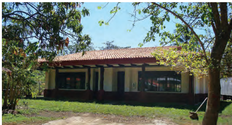
EARTH-La Flor's energy-efficient buildings are inspired by the traditional architecture of the Guanacaste region.
